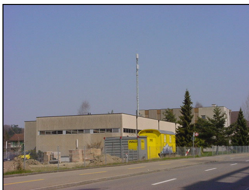
figure 12-22: View of the KONI installation
