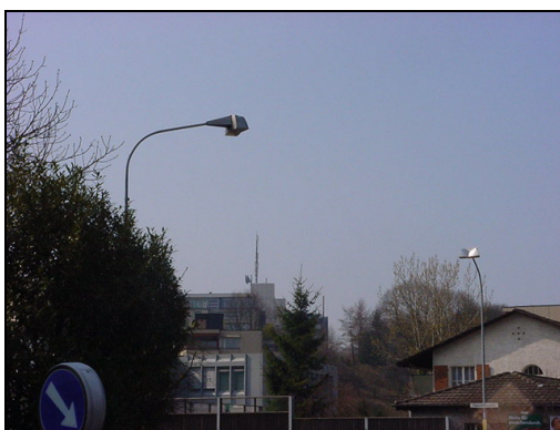
figure 12-8: View of the ITTI installation
