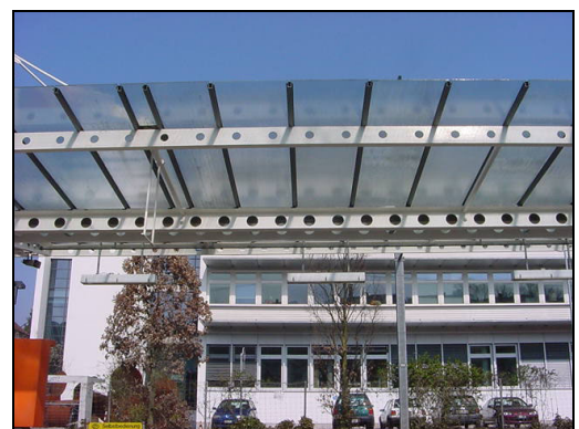
figure 12-9: View of the BUWAL building where the indoor measurements were performed
