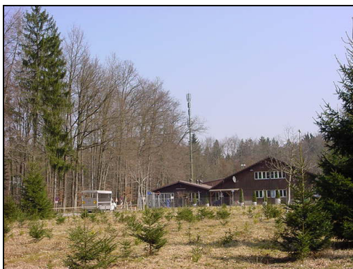
figure 12-5: View of the BEFH installation
